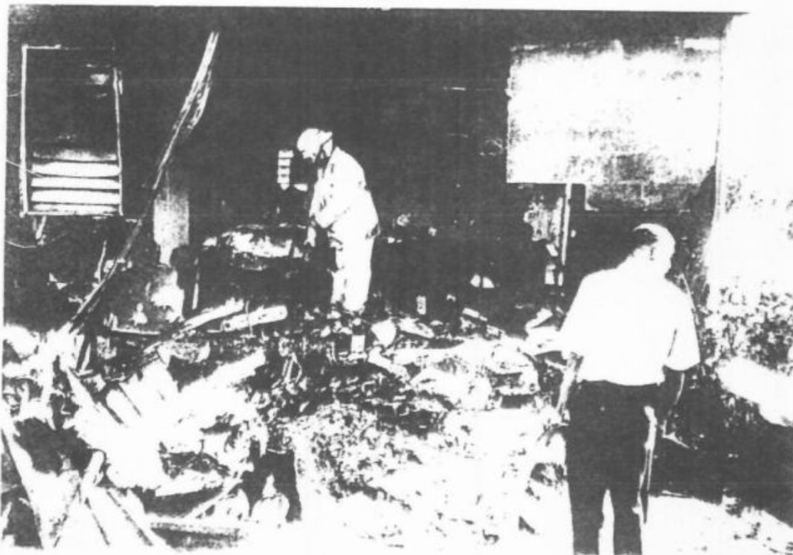
House wall destroyed by aircraft impact
